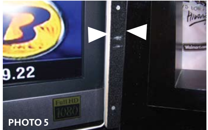
If the TV is to be flush-mounted, a thin strip of wood trim can be stained and attached to the exposed face with hook-and-loop fastening material.
