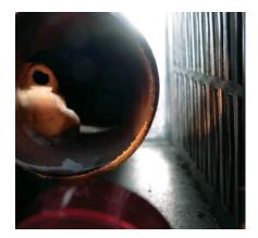
Clear the furnace's intake and exhaust vents of any debris that would restrict fresh air from entering the combustion chamber and exhaust from exiting it (above). A main blower wheel weighted down with dust and dirt (right) may be too heavy to turn with adequate speed, thereby keeping the furnace from firing. Check the interior air ducts for blockages, such as rodent nests (opposite), that could keep the heated air from warming the motorhome.
